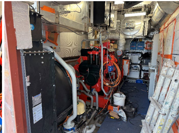
Heat recovery system cooling water harbour / emergency generator
