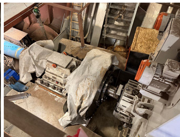
Flexible linkage between the engine and drive shaft has been installed.
