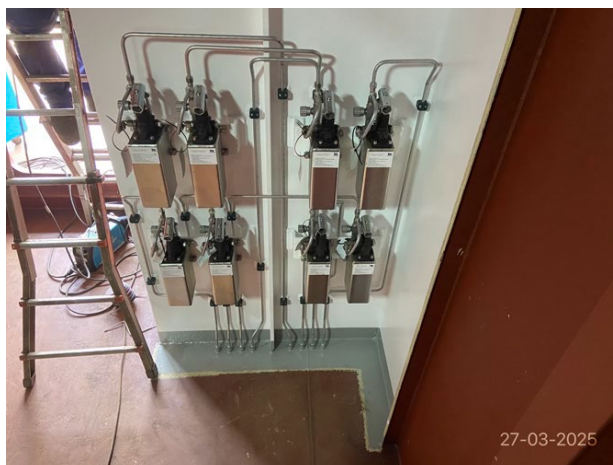
Sliding door emergency controls
