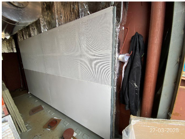
Emergency generator room insulation
