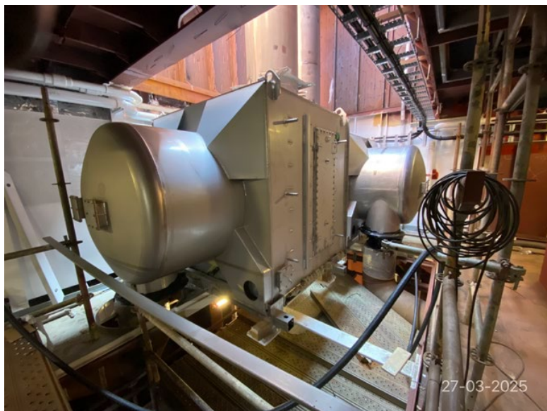
DPF and leads SCR for the generators
