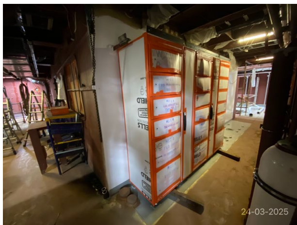
Pump starter lockers (MCC)
