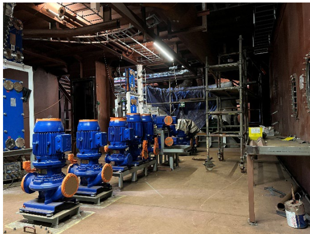
Pumps located in the engine room and bow thruster room.
