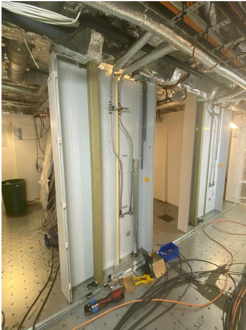
*The cabin partition bulkheads, with the various connections and cables visible.*
