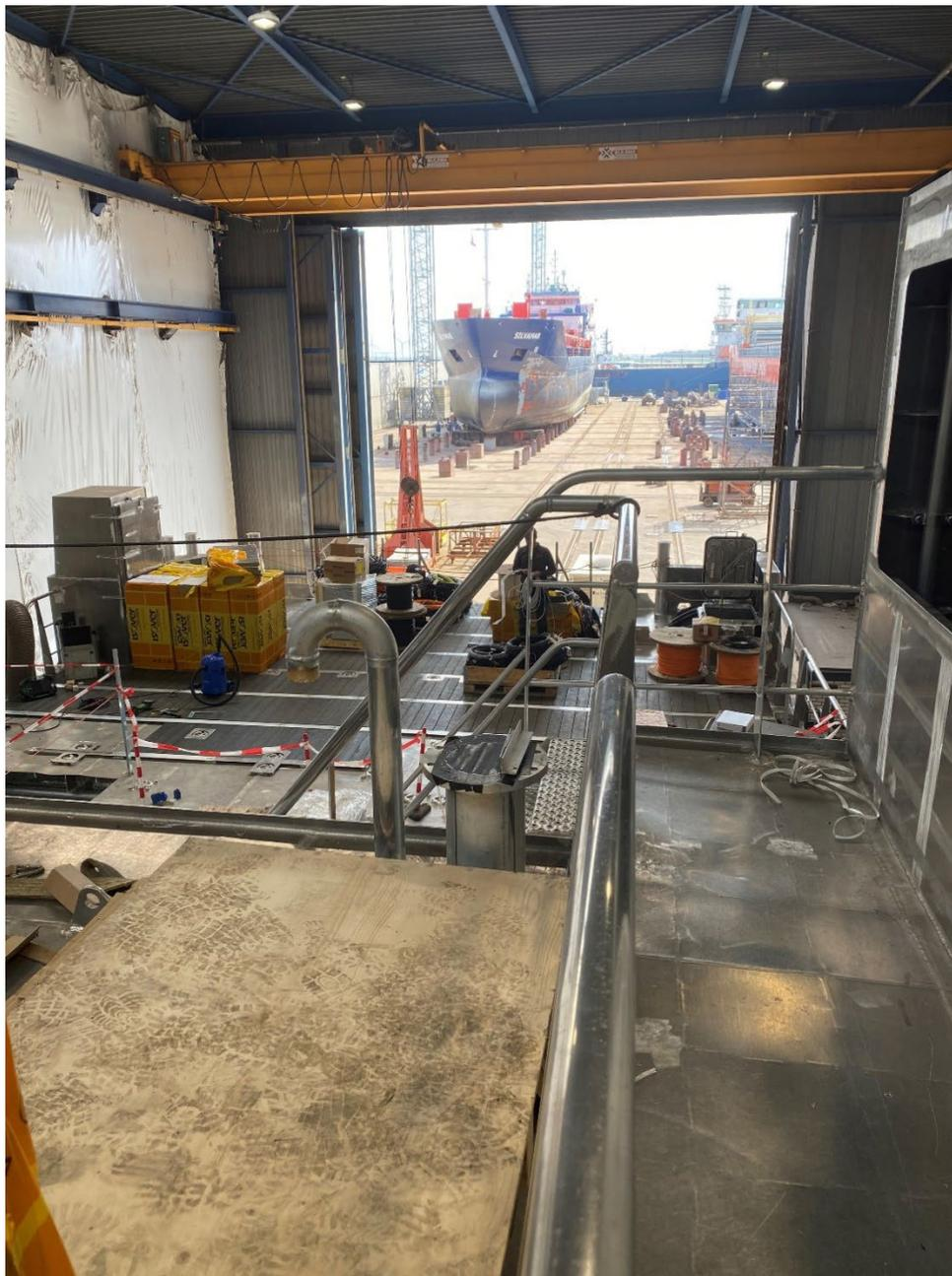
*View aft from the bridge, showing the working deck where builders are fitting the synthetic deck panels. The repair yard at Damen is visible through the open bay doors.*
