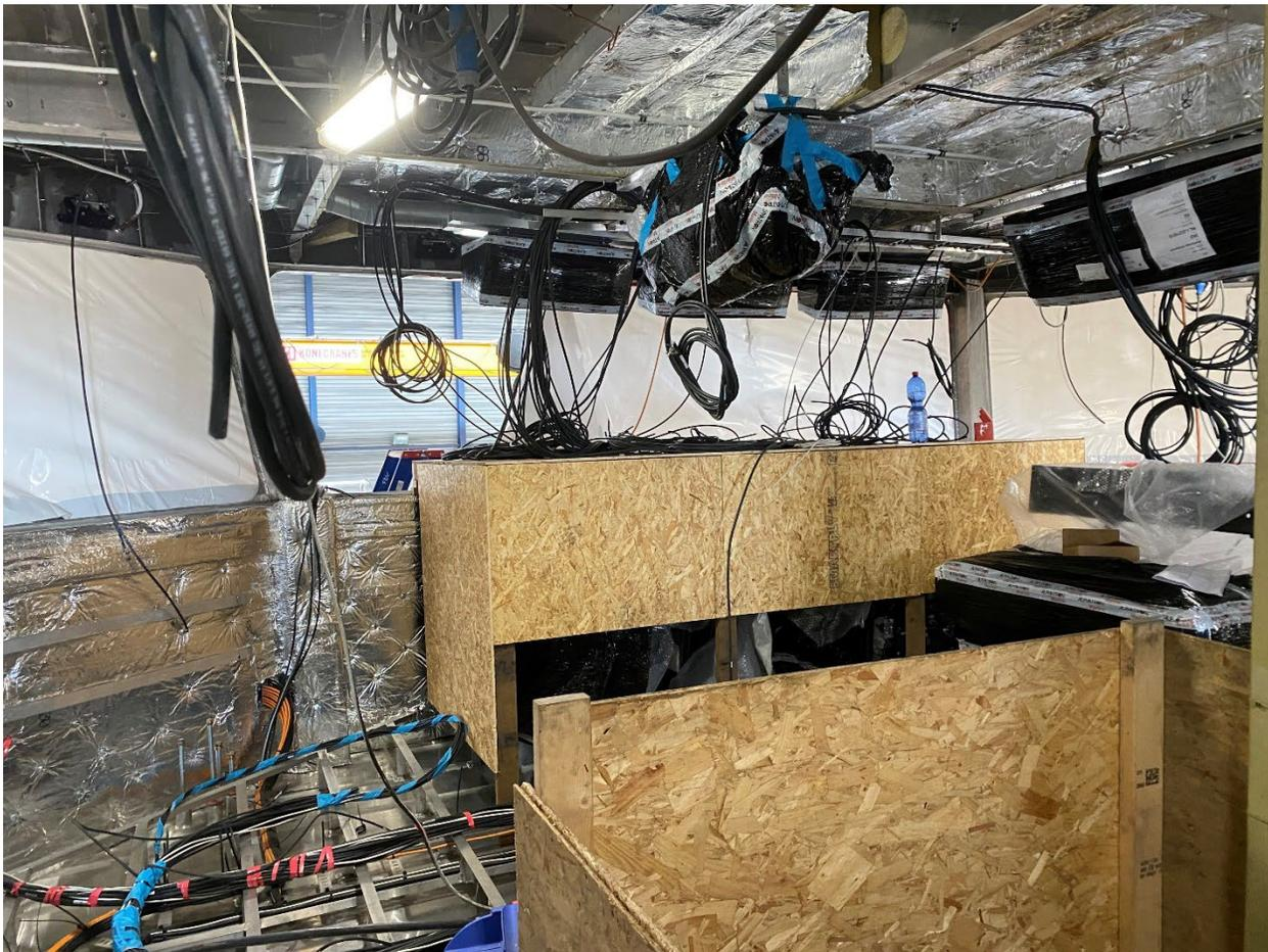
*The wheelhouse, showing the various consoles. The consoles fitted to the deck will be protected with a housing.*
