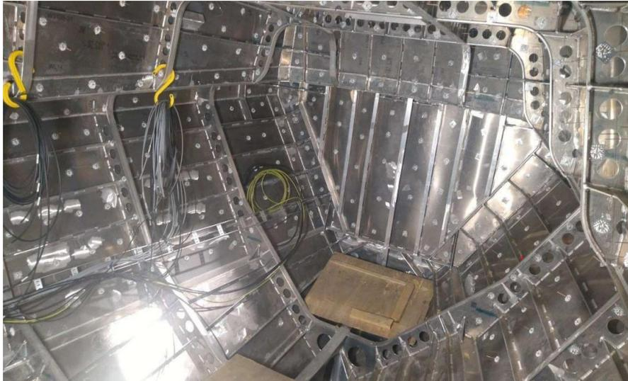
Day cabin with galley, showing pins fixed to the aluminium for attaching the insulation. ©NGS
