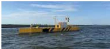
Prior to tethering, dedicated research was carried out aboard our own research vessel *Navicula* in finding the optimal location for BlueTEC. The challenge: staying away from navigational channels, avoiding the high frequency island ferry and achieving maximum power output. Our calculations showed tides could, in theory, produce at most 90 MWh per year, and in practice the turbine is currently already churning out up to 40% of that.
