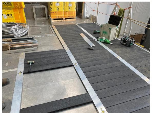
The protective synthetic panels on the aft deck are installed and secured between aluminium strips.
