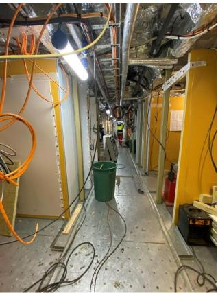
The first partition bulkheads for the crew and passenger cabins have been installed on the false deck below decks. ©FH
