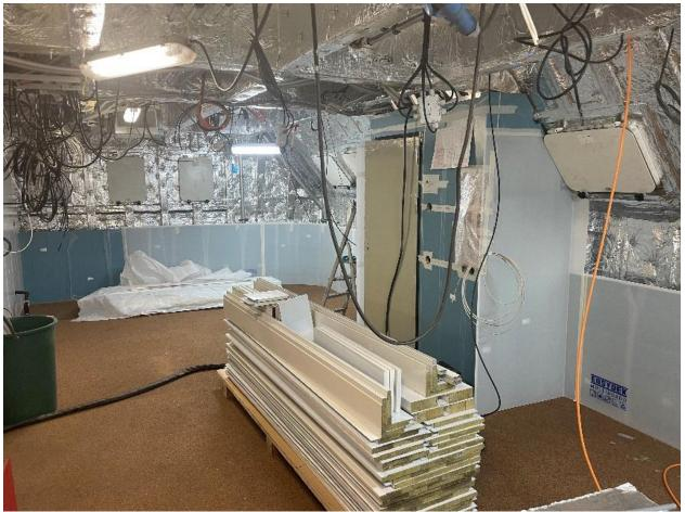
The messroom, with the noise- and vibration dampening deck cover. The first partition bulkheads have already been installed. ©FH
