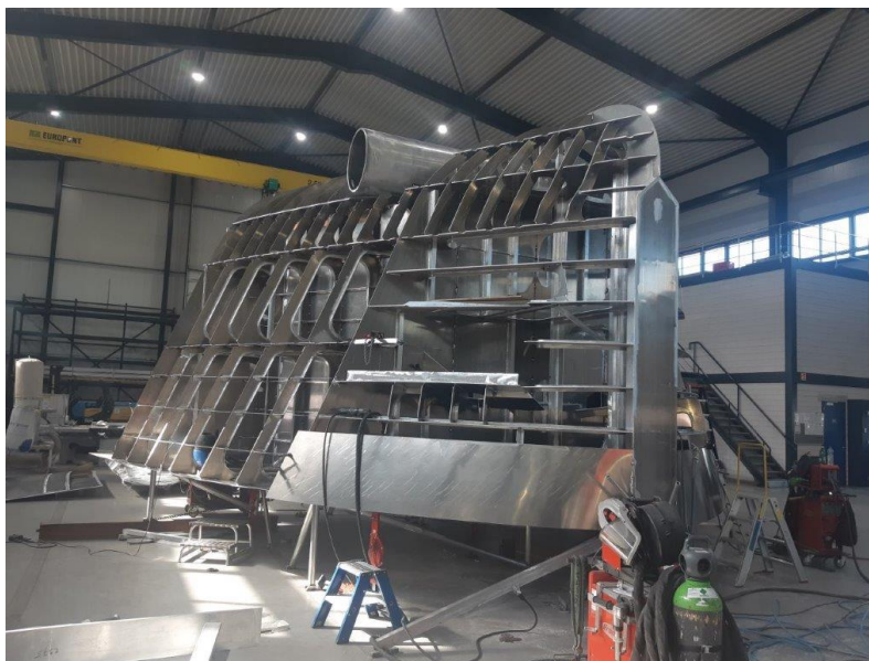
Bow section 510 at Bloemsma in Makkum, with the tunnel for the bow screw clearly visible.
