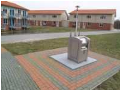
Underground refuse containers
