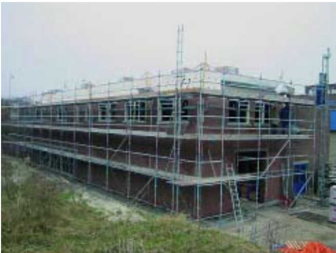
The new workshop-space and offices of Marine Technology Mechanical
